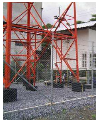
Fence Installation Completed
